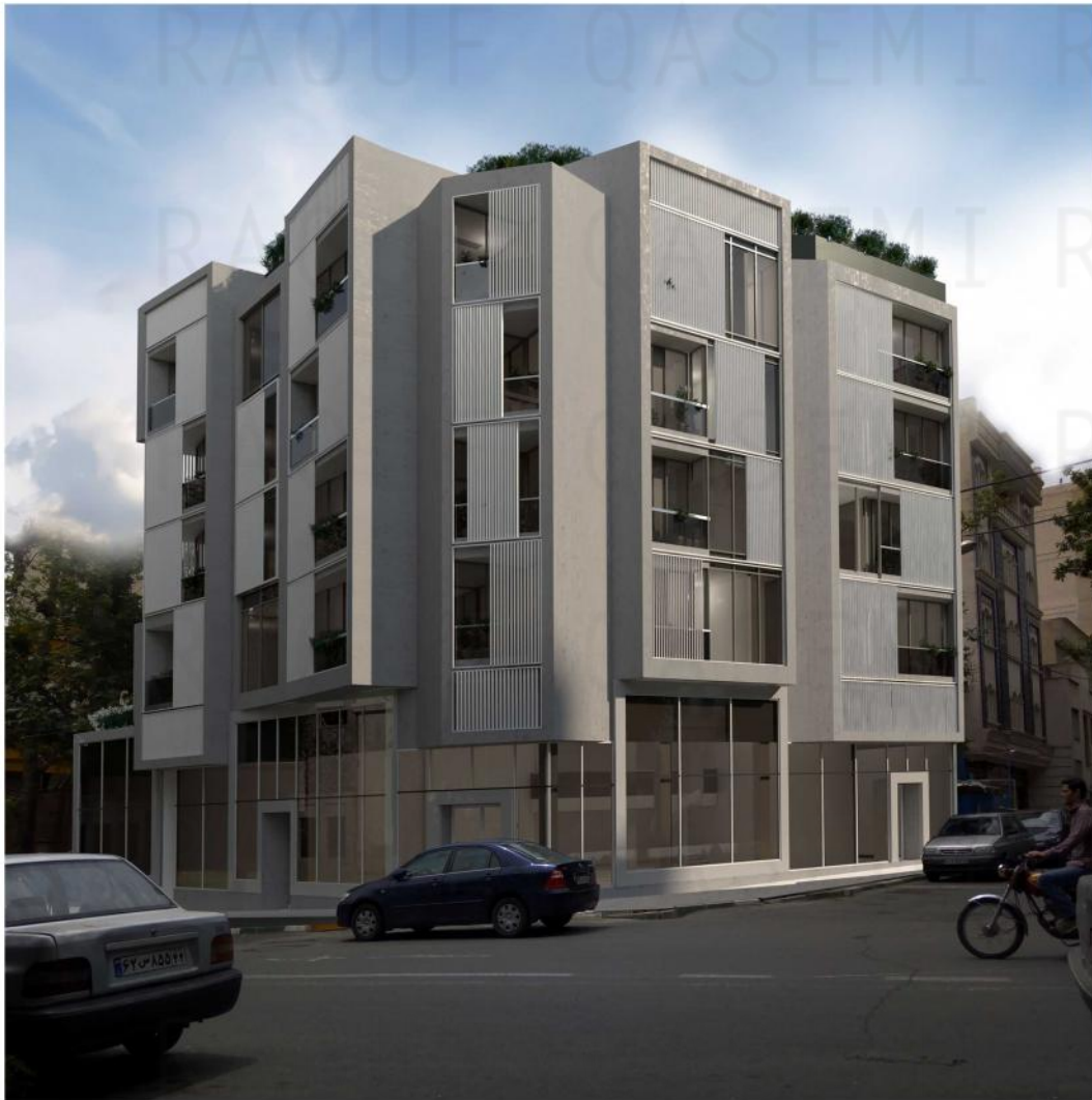
Mojdeh OFFICE BUILDING -2018
